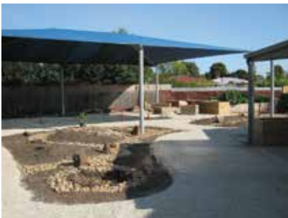
The project nears completion.
